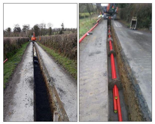
Plates 2 & 3: Typical Trench Construction
