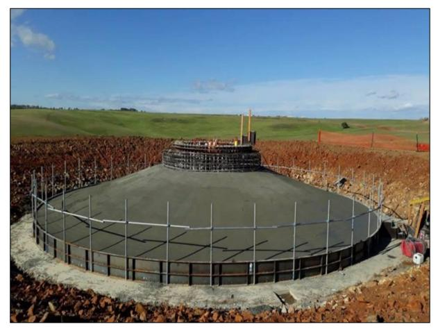
Figure 3.5: Typical Turbine Foundation
